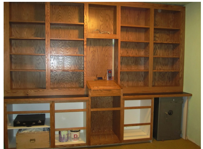
Tyler's Room (work in progress)
